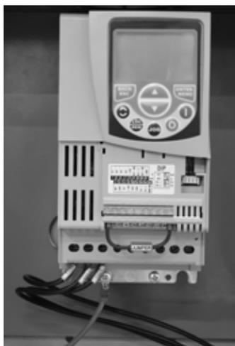
Figura 6A - Bornes com jumper
